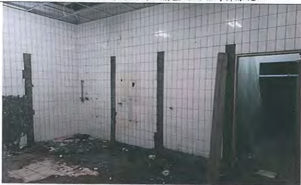
3樓待勤盥洗室磚造隔間牆拆除施工
