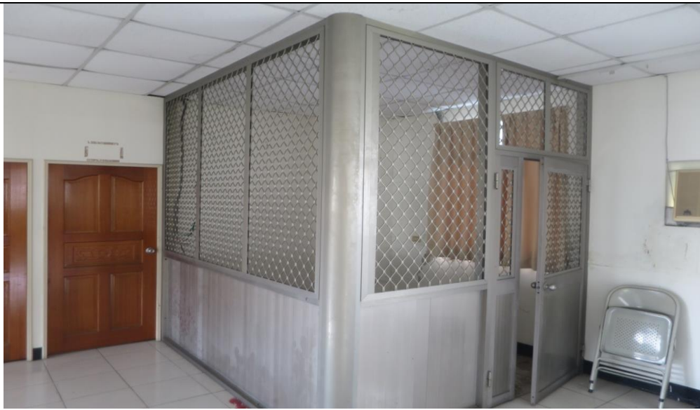
盥洗室施工前
